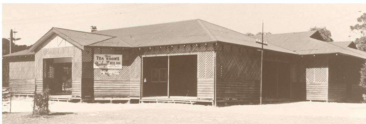
A variety of P1 Huts repurposed and reconfigured as the Rottnest Tea Rooms roughly on the site of the current Dome Coffee Shop
