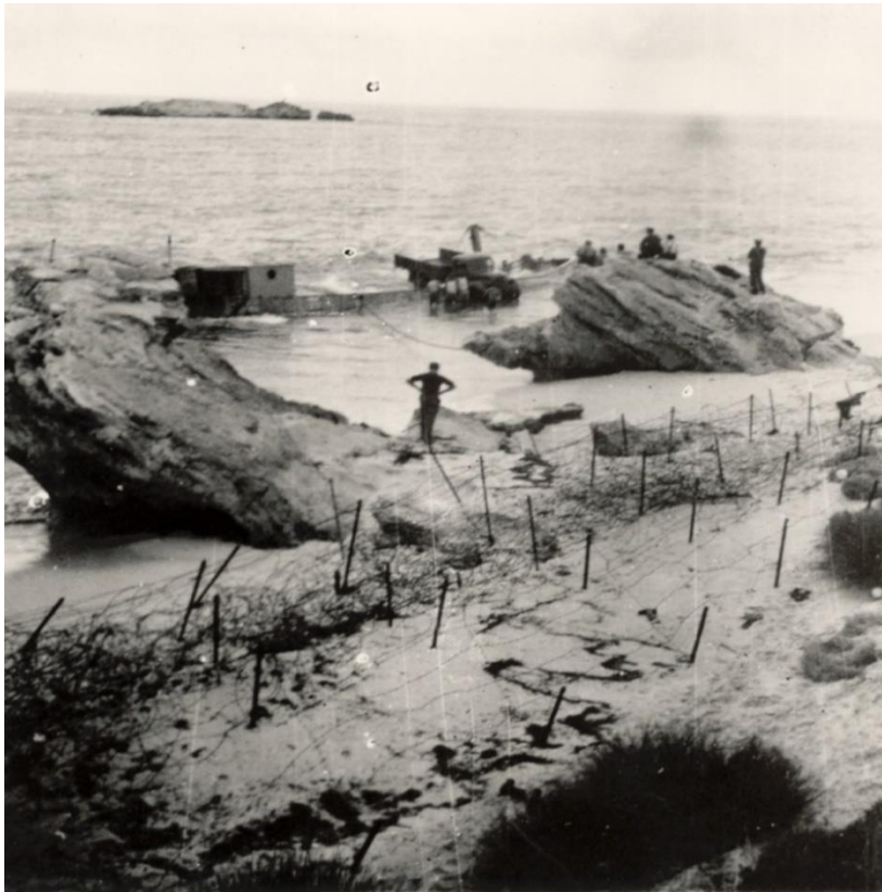
Beach defence fence – appears to be double height concertina with double apron. Salvage of truck from Uribes in Thomson Bay. Cut down Phillip Rock is visible in the background to facilitate clear sweep pattern for Bickley Point searchlight. The Uribes was wrecked in 1942.
