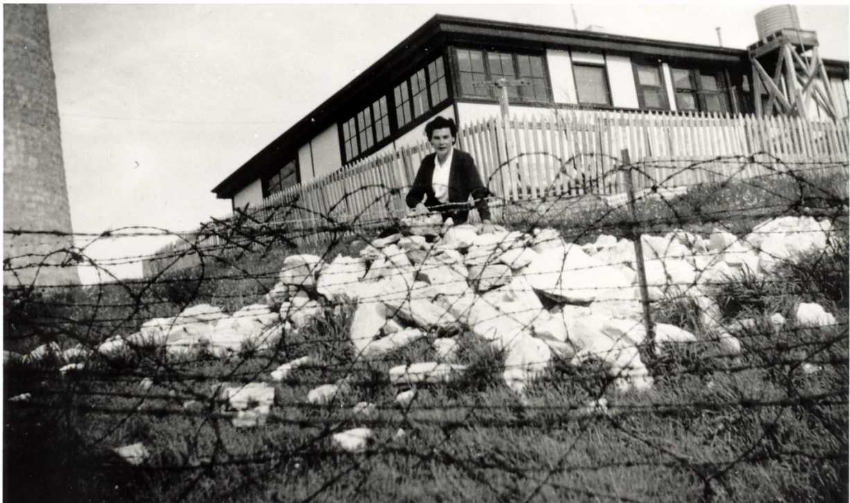
WRAN's Quarters at Signal Ridge / Wadjemup Hill, Single stand concertina with single apron.
