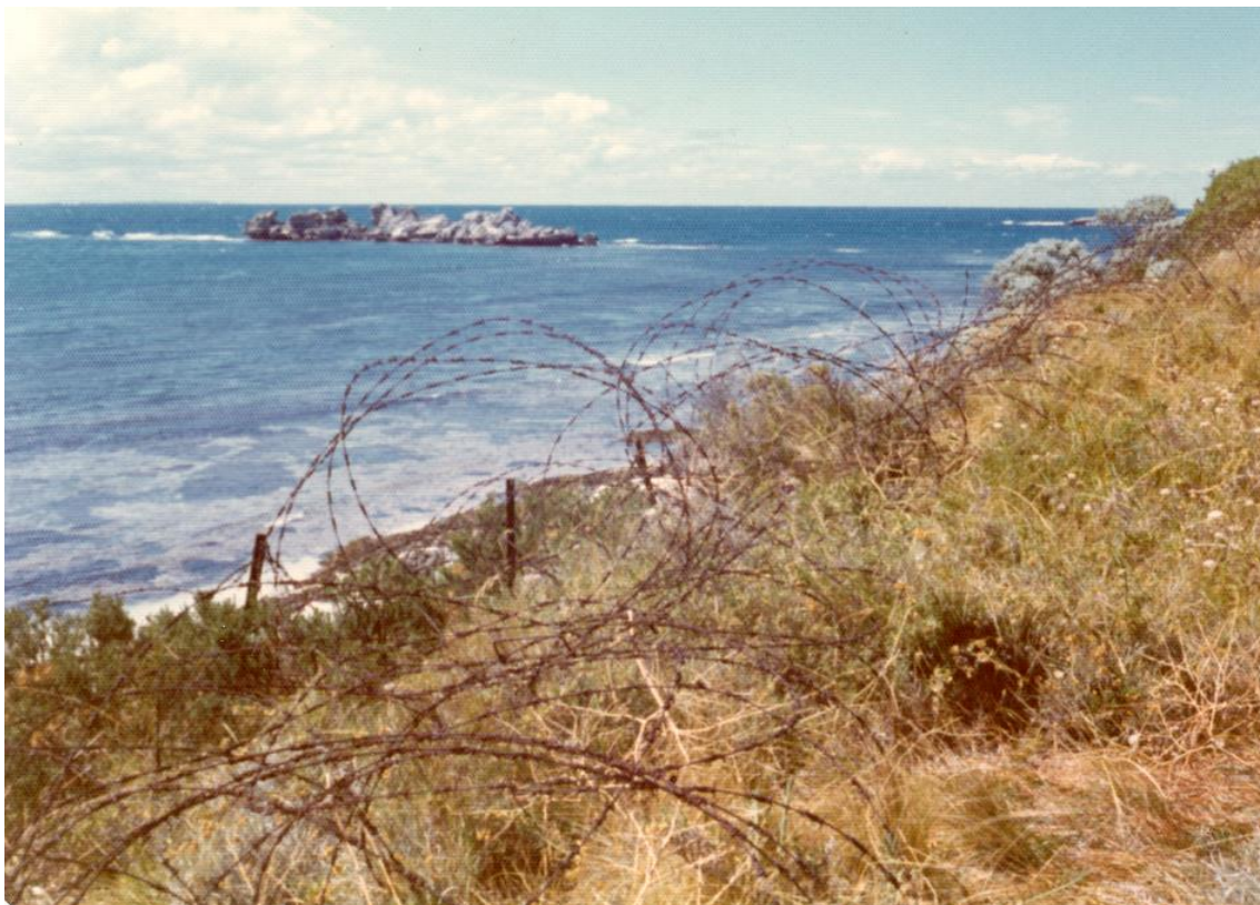
Close in defensive fence – Bickley Battery – Appears to have been double height concertina with single apron
