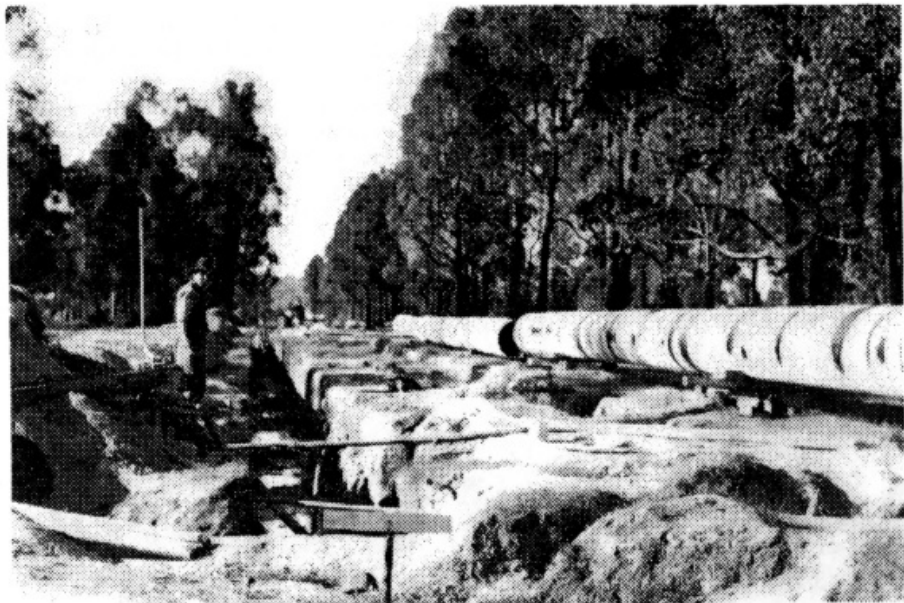
Photo: Relaying pipes through Chidlow 1938 (Photo courtesy West Australian Newspapers)
